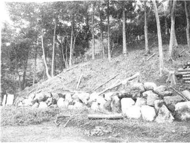
写真-3 箱根町の対象斜面 Photo 3 Survey slope at Hakone town
